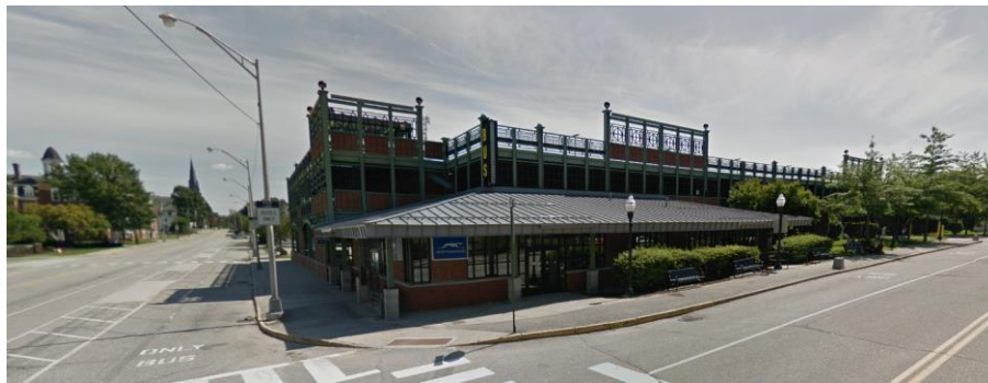
Figure 5 Oak St. Transit Hub (Source: Google Maps)
